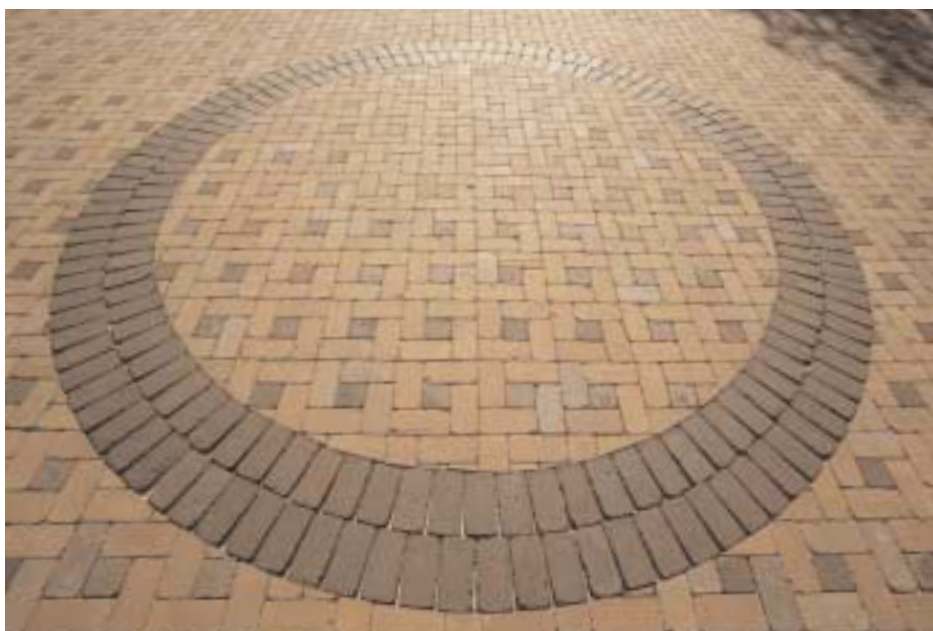
One of the company's most intricate installations was this tumbled clay, brick driveway and path in two patterns — a modified basket weave and herringbone. Clay bricks take longer than pavers to install, and this driveway at The Tradition took about a month.
